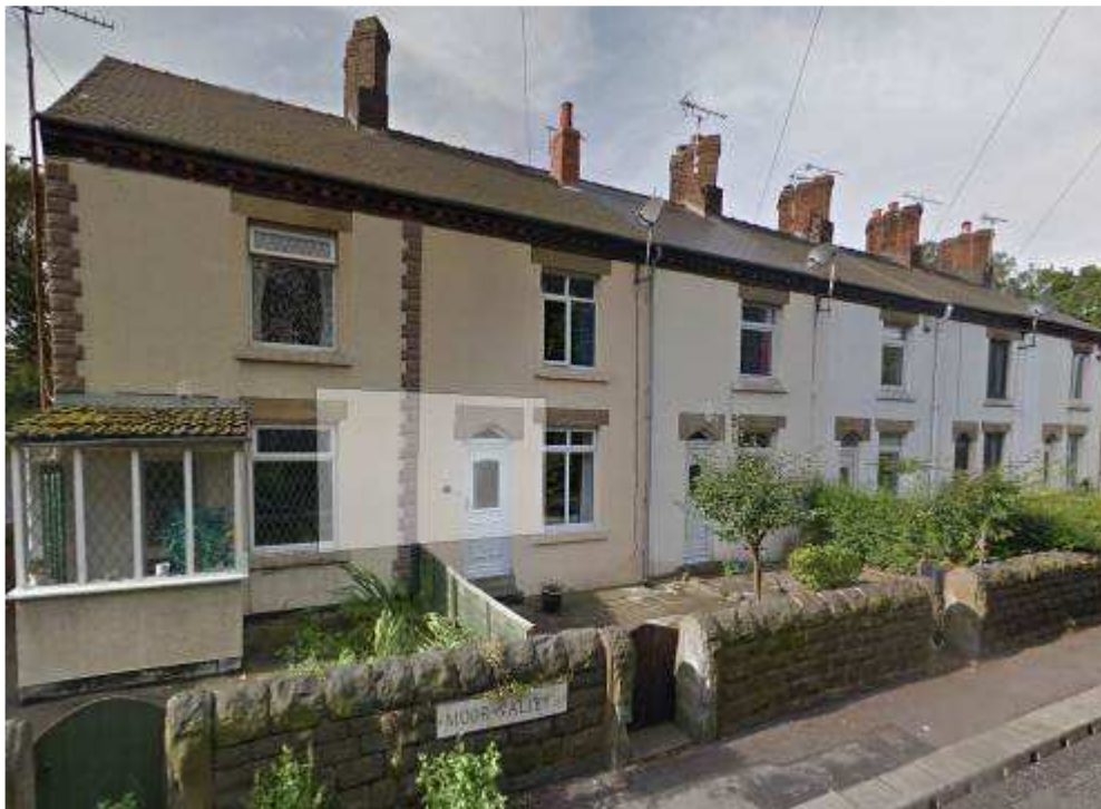
Photograph 3 showing the boundary treatments of the other properties in the terrace.
